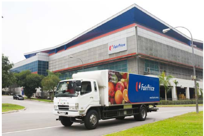
Fresh Food Distribution Center
